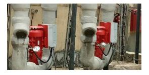
Armstrong maps each individual pump's hydraulic, motor and inverter variations at the factory, to achieve exceptional accuracy throughout the flow range. With this calibration, Armstrong Design Envelope pumps also serve as flow meters, providing reliable system flow data (+/- 5%). The testing ensures optimal performance efficiency at start-up, and Armstrong's Pump Manager helps maintain and extend efficiency throughout the pump's operating life.
